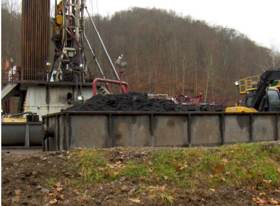
Drill cuttings on a well pad in the US ( https://www.frackcheckwv.net/2014/03/11/wv-legislature-will-need-a-special-session-to-complete-marcellus-landfill-regulations/ )
